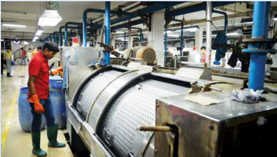
A large washing plant financed by Dhaka Main Branch
